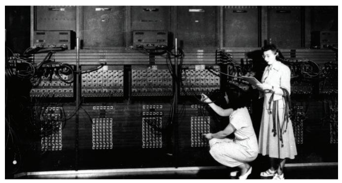
Two programmers wiring the right side of the ENIAC with a new program.
